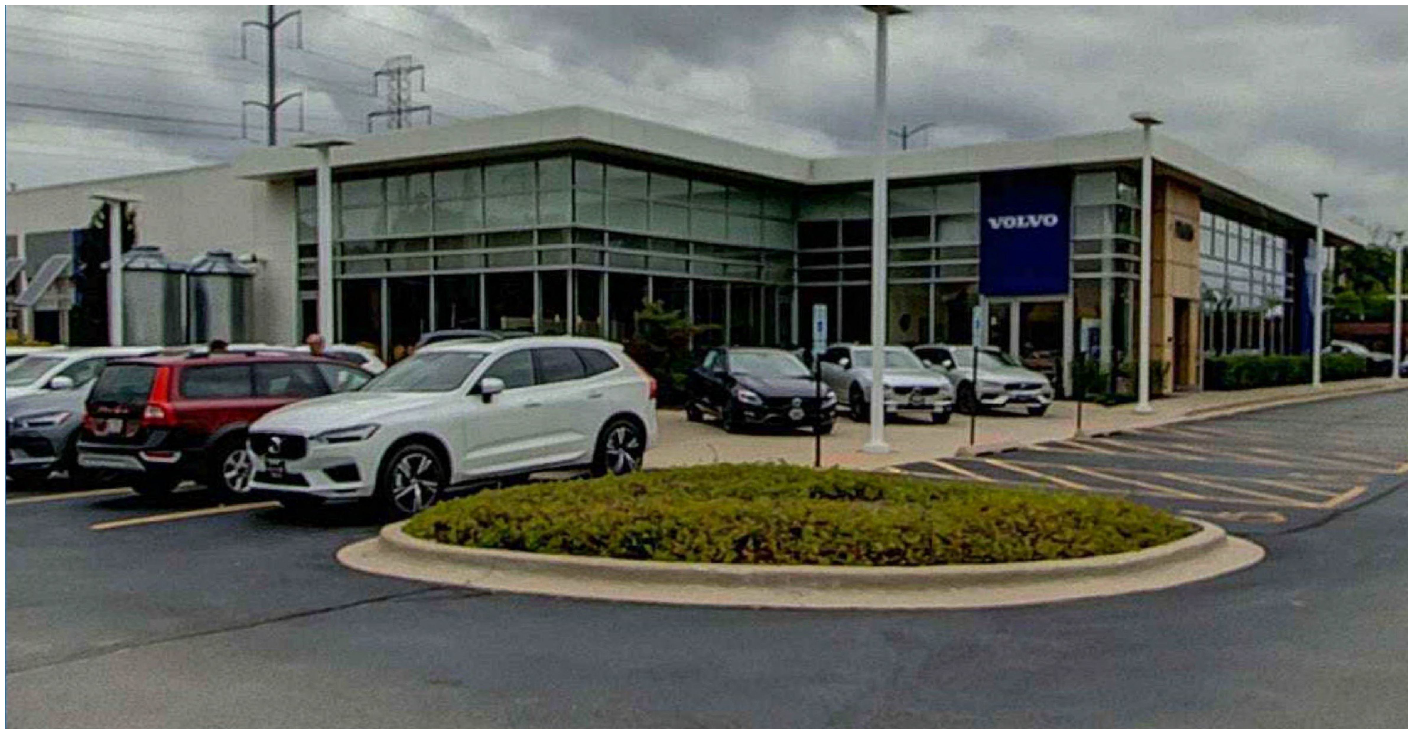
Existing Image | East Overall View NTS
