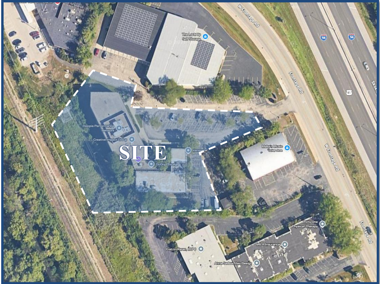
Aerial View of Site
