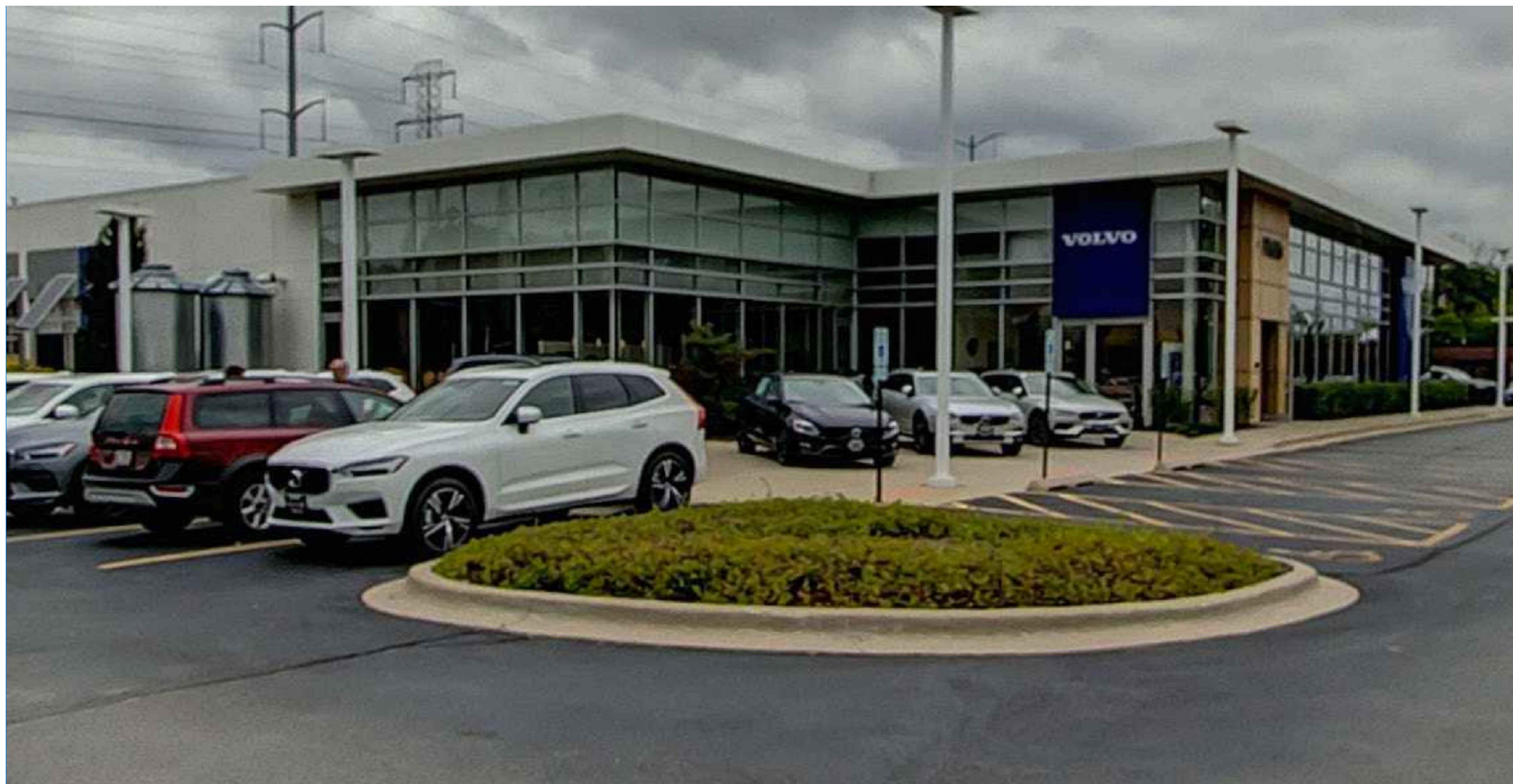
Existing Image | East Overall View NTS
