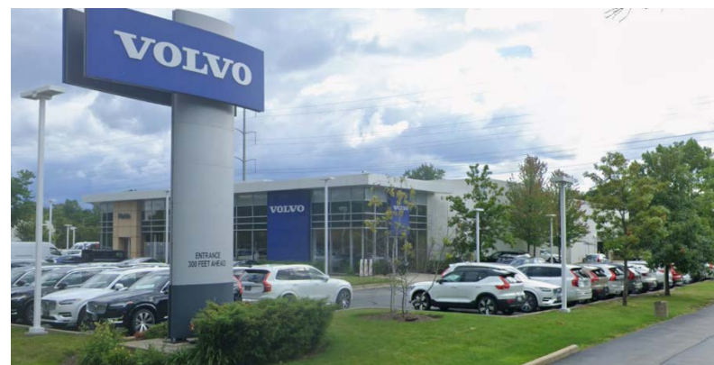
Figure 8 Streetview of the northeast side of the existing Volvo building
