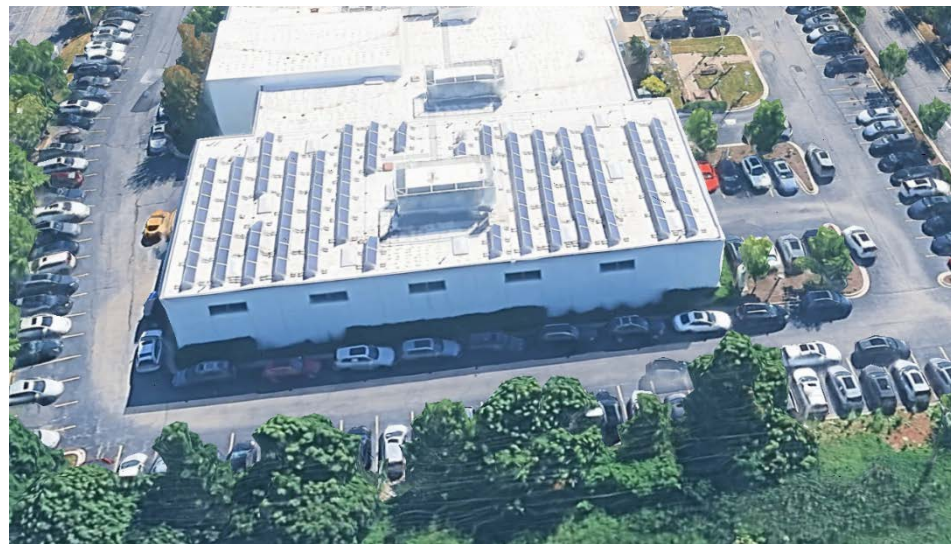
Figure 6 aerial view of the existing west side of the Volvo building
