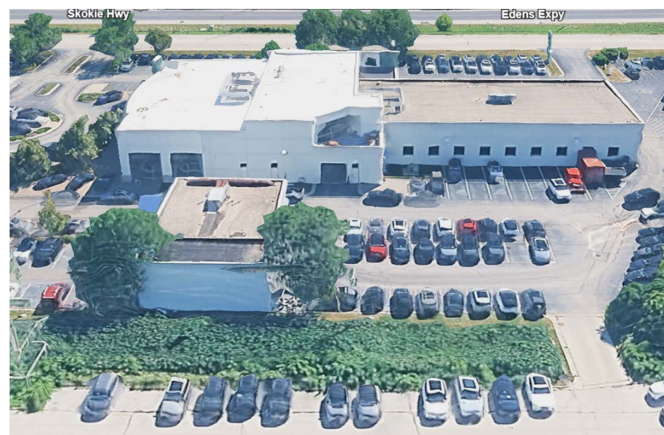
Figure 3 aerial view of west side of the existing carwash with the JLR dealership behind it
