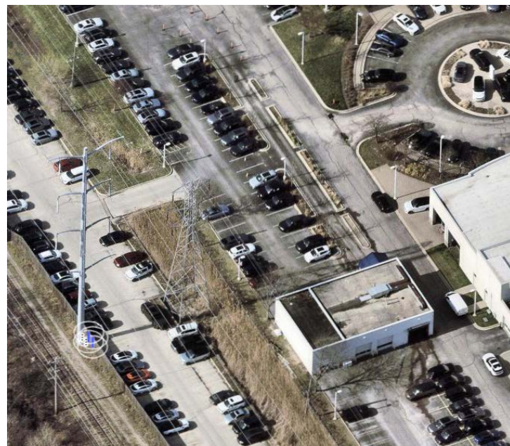
Figure 2 aerial view of the southwest side of the existing carwash
