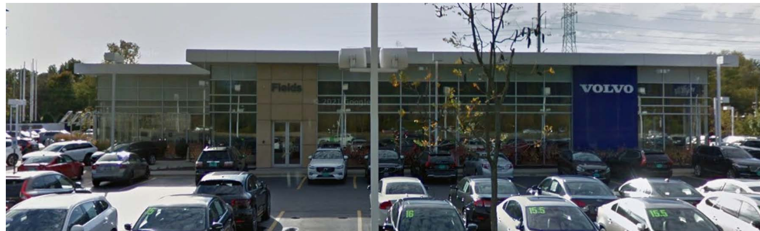
Figure 7 Streetview of the east elevation of the existing Volvo building (the left south side will be the location of the expansion for the showroom)
