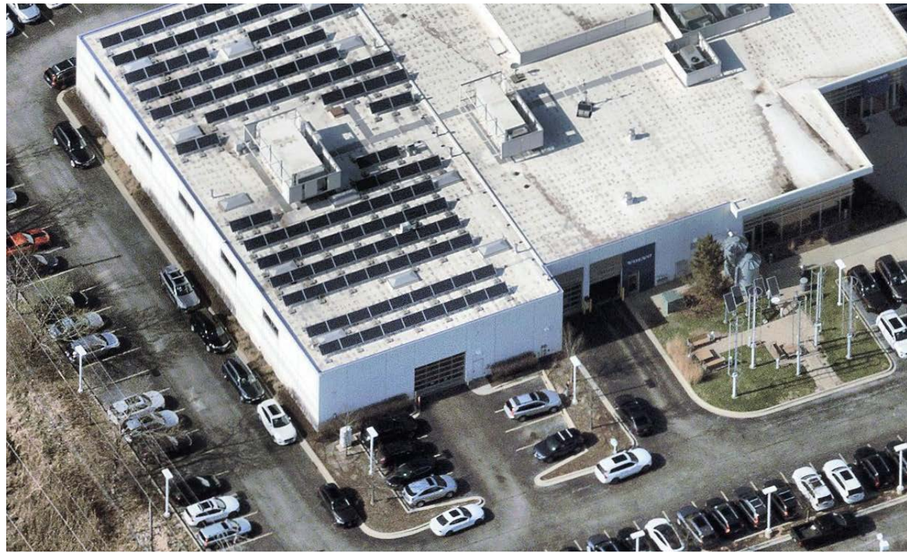
Figure 4 aerial view of the southwest side of the existing Volvo building
